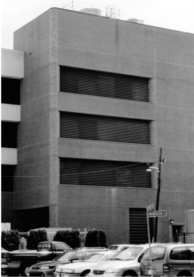
Figure 15.4 Reentry problems caused by proximity of loading dock to HVAC intakes at side of building.
