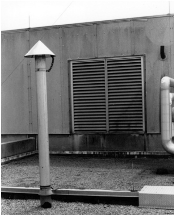
Figure 15.2 Actual reentry situation. Design flaws include insufficient stack height, proximity of stack to HVAC intakes and the presence of a rain cap.
