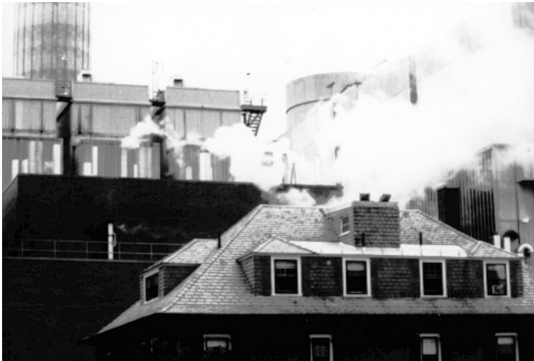
Figure 15.6 Effect of complex wind pattern on stack exhaust. Three photos taken within minutes of each other show widely varying flow patterns.
