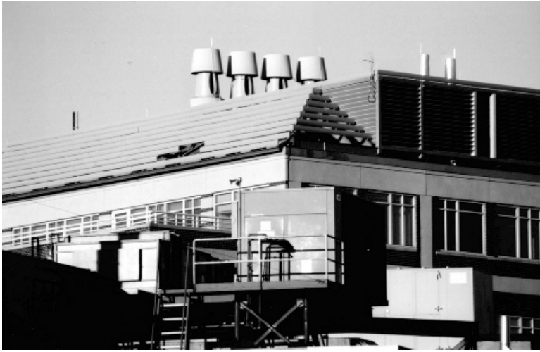
Figure 15.13 Stacks that entrain ambient air into the exhaust.
