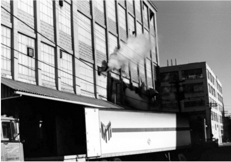
Figure 15.11 Side exhaust from side of building may lead to reentry condition.
