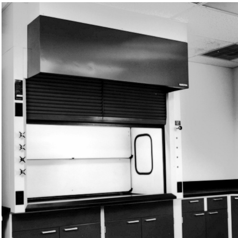
Figure 7.10 A well-designed auxiliary air supply hood with a bypass detail. The outside air is introduced through a canopy designed to provide a laminar flow pattern that blankets the hood face and blends with room air as it enters the hood. The hood is designed to provide air at room temperature during the heating season; unconditioned air is supplied during cooling periods, thereby saving air-conditioning costs for the air supplied through the canopy. An additional advantage is less well known. When a person stands in front of a laboratory hood, a slight negative pressure is created between his or her body and the hood, causing turbulence and loss of contaminant from the hood. The auxiliary air supply fills this space, eliminates turbulence, and improves containment efficiency. (Courtesy of Fisher Hamilton Industries LLC.)
