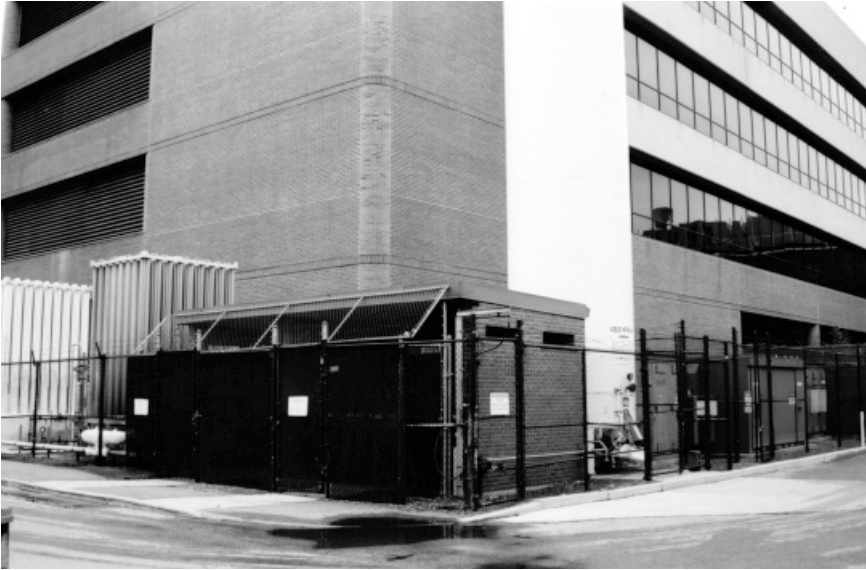
Figure 15.3 Reentry problems caused by near-ground-level exhaust and HVAC intakes at side of building.
