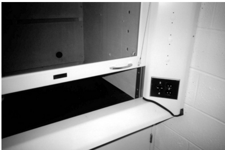
Figure 7.7 The turbulent eddies at the hood corner posts can be minimized by modifying the hood inlet geometry. An ideal corner post would have the form of a bell mouth. In practice this is frequently approximated with a simple angled detail, which is inexpensive to fabricate and install, but effectively minimizes the entrance eddies and improves contaminant control at the entrance to the hood. Although the same simple geometry used on the corner posts could be used to improve the entrance geometry at the front lip of the work surface, a more effective approach is the displaced airfoil. This element breaks turbulent eddies, provides a well-defined airflow path to sweep the hood work surface when the sash is down, and may be used to define the minimum working distance from the face of the hood. The space between the work surface and the airfoil should be large enough so that the operator can pass through tubing and electrical cables.
